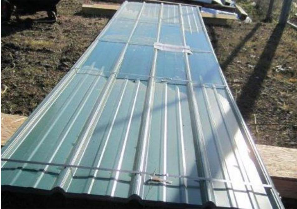
Insufficient support in the center of long panels allow “Bowing” or “Sagging” that traps water in the center of the panel length.
